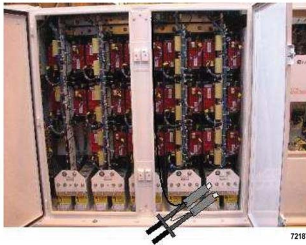
FIGURE 00-10. APPLICATION OF GROUNDING STICKS TO CAPACITOR TERMINALS
